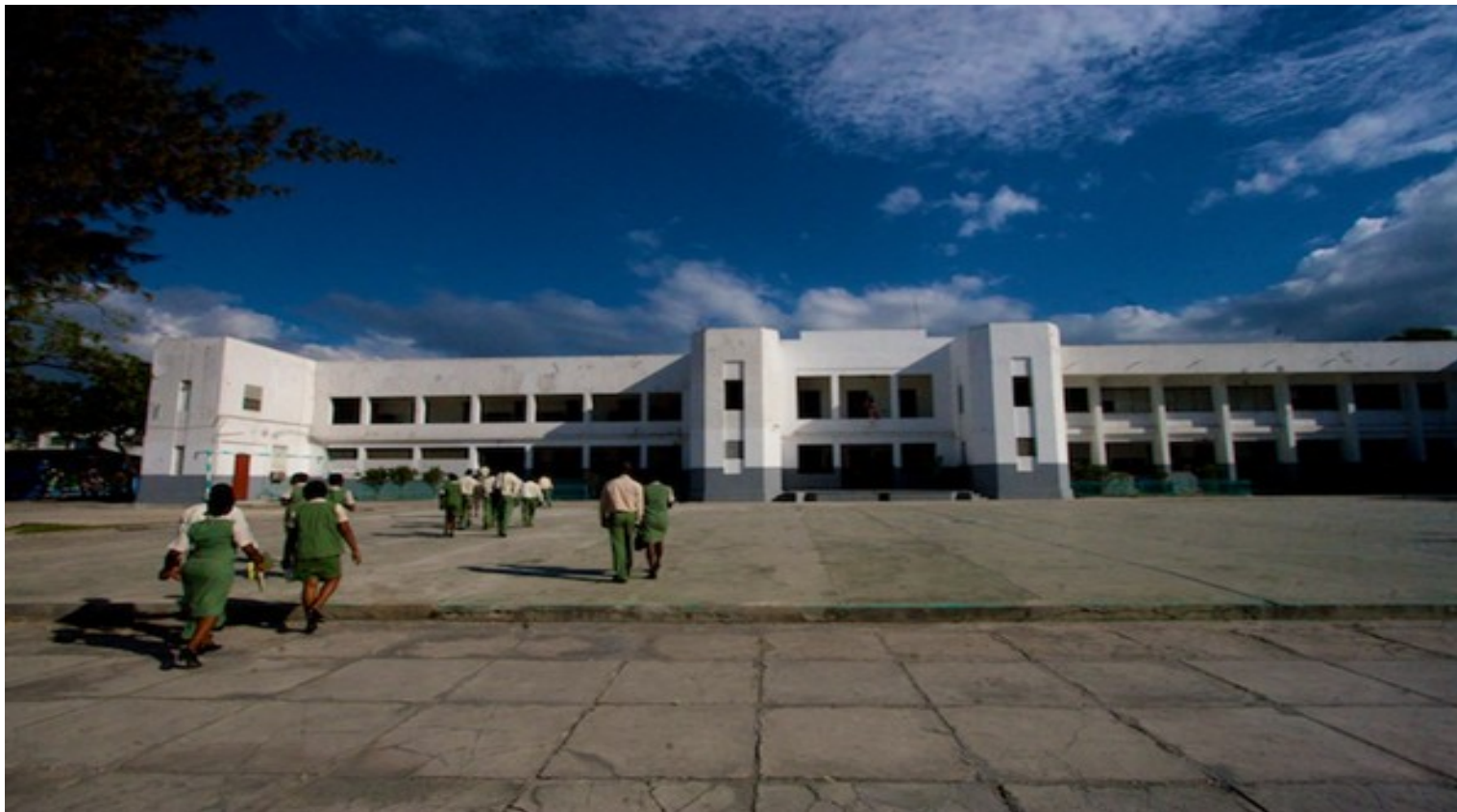
ENAM main building prior to the 2010 Earthquake
